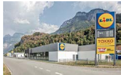
24. Flums, Lochrietstrasse 27/27a/27b/29
